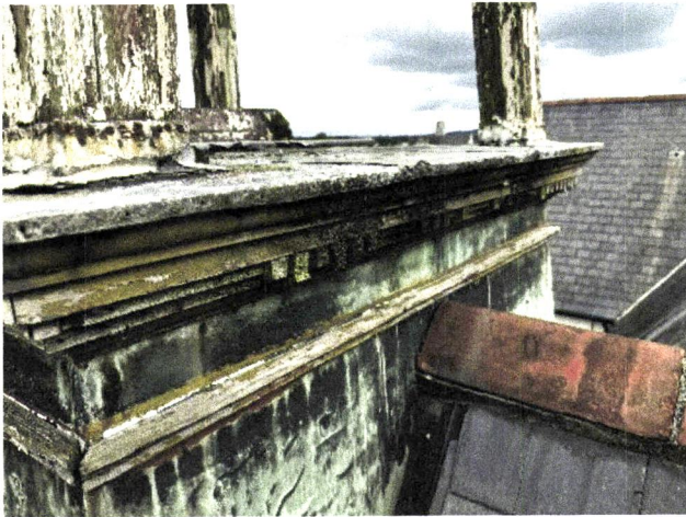
Photograph 17: Single section of lower decorative element that could have moulding taken for reinstatement onto other three posts
