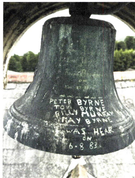
Photograph 8: Inscriptions on bell from potential previous works / repairs
