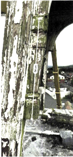
Photograph 17: Single section of lower decorative element that could have moulding taken for reinstatement onto other three posts
