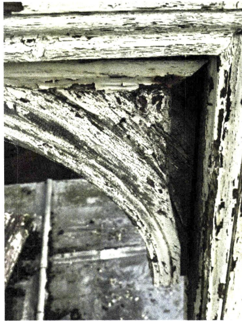
Photograph 12: Close up of decorative timber element corner detail
