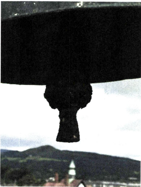
Photograph 7: Seized hammer to bell
