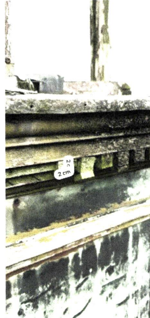
Photograph 22: Timber feature on dais walls over copper cladding
