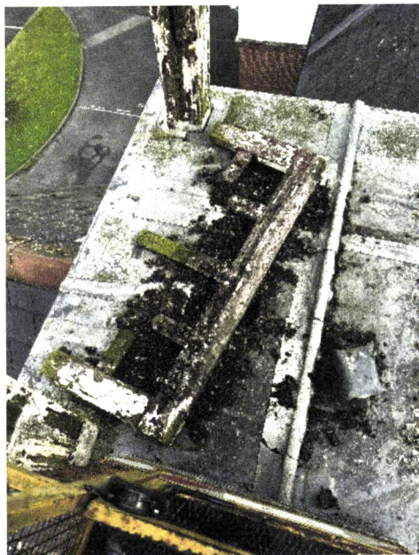
Photograph 11: Original section of decorative timber skirt to bell tower
